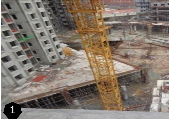
C, D,E South Side Podium Shuttering and Reinforcement in Progress
