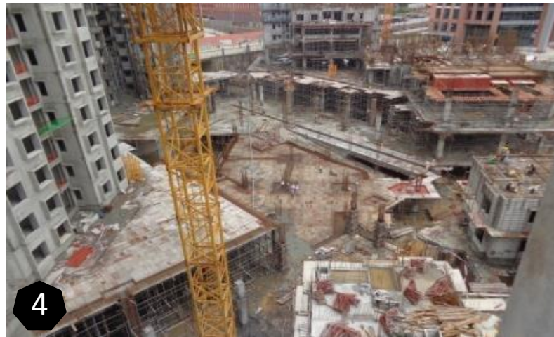
Tower A Podium Area Slab Shuttering, Reinforcement and PCC in Progress.
