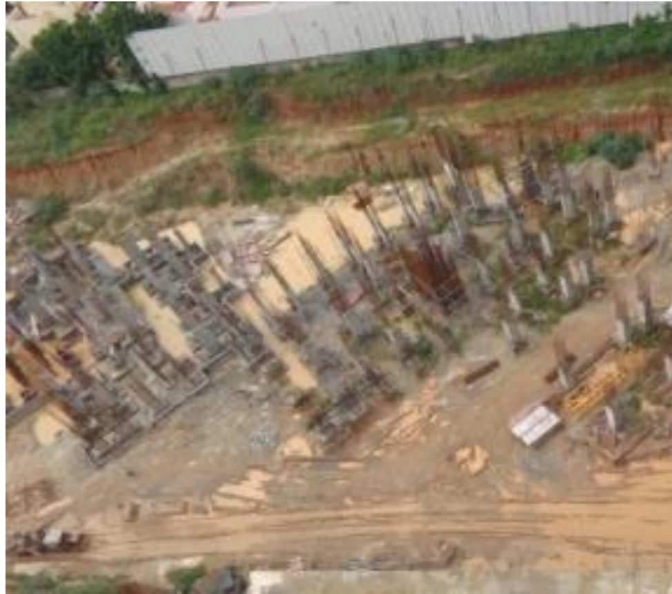
TOWER L : Lower Basement Column Casting Works in Progress.
