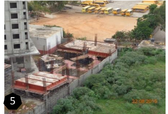
F & G South west Podium Slab Shuttering Works in Progress.
