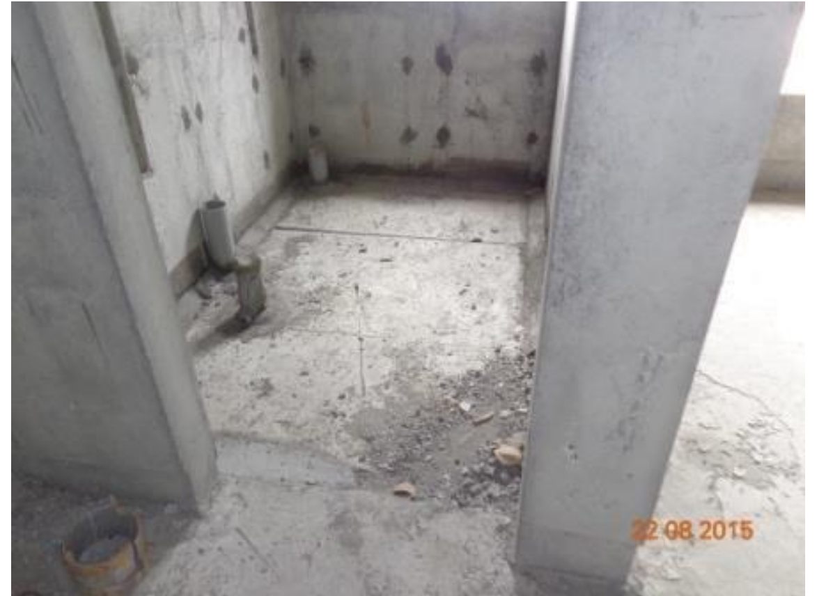
TOWER F : Above Terrace works and Toilet Bore Packing Works in Progress
