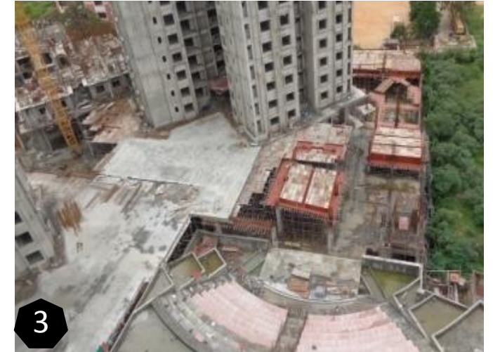
F Podium North Side Slab Shuttering ,Reinforcement and Concrete in Progress.
