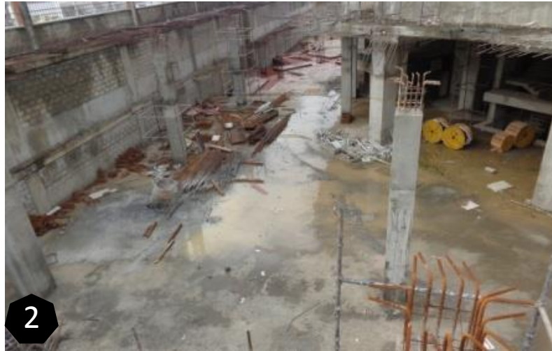
A & B Podium North Side Shuttering in Progress
